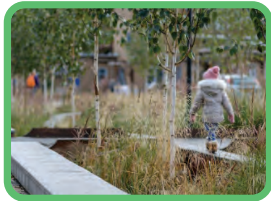
Vegetated SuDs feature incorporated in surrounding landscape design increases ecological value and provides visual amenity.
