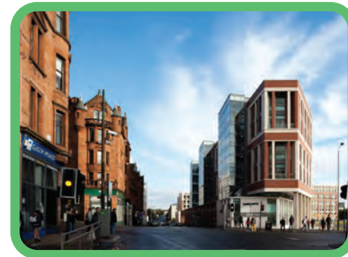
Colour of new offices responding to context
