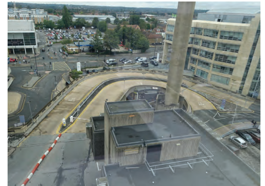
Fig. 29 - Existing ramped access & HTC building
