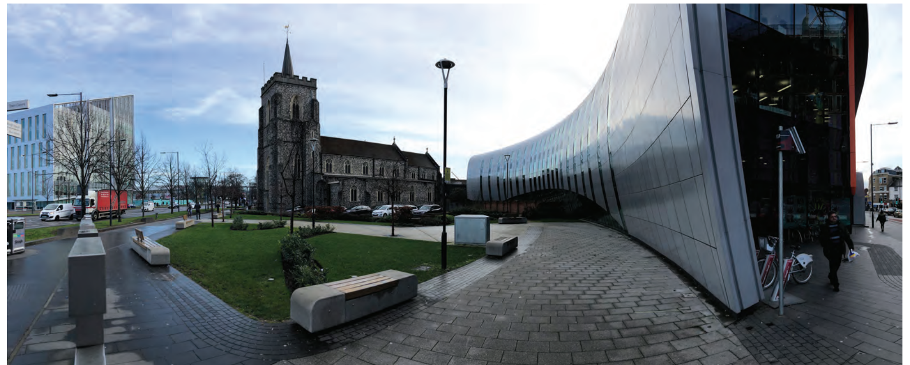
Fig. 11 - Photograph of Church of Our Lady Immaculate and St Ethelbert and Curve building
