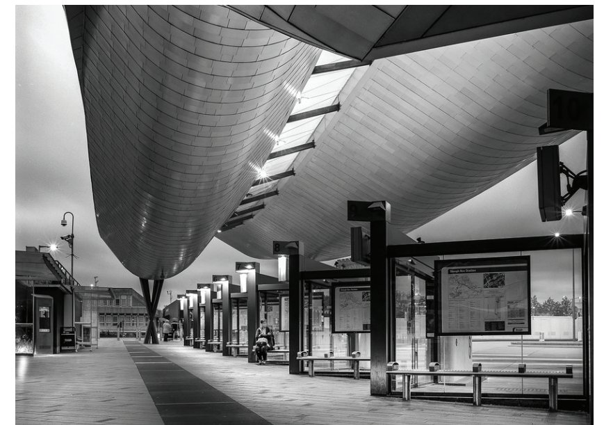
Fig. 21 - Photograph of Slough Bus Station
