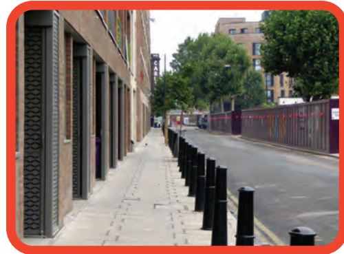
No separation between pavement and residential entrances
