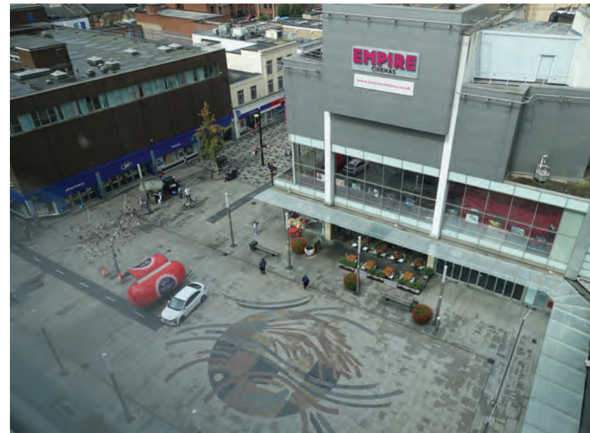
Fig. 28 - Very few natural features are incorporated in the available areas of public realm on the site
