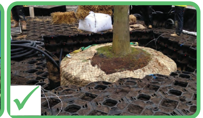
Fig. 71 - Cellular systems used in paved areas
