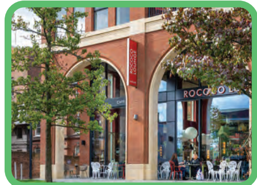
Clearly defined ground floor retail
