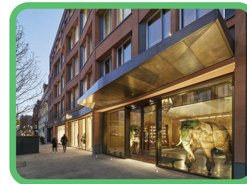
Canopy over residential entrance
