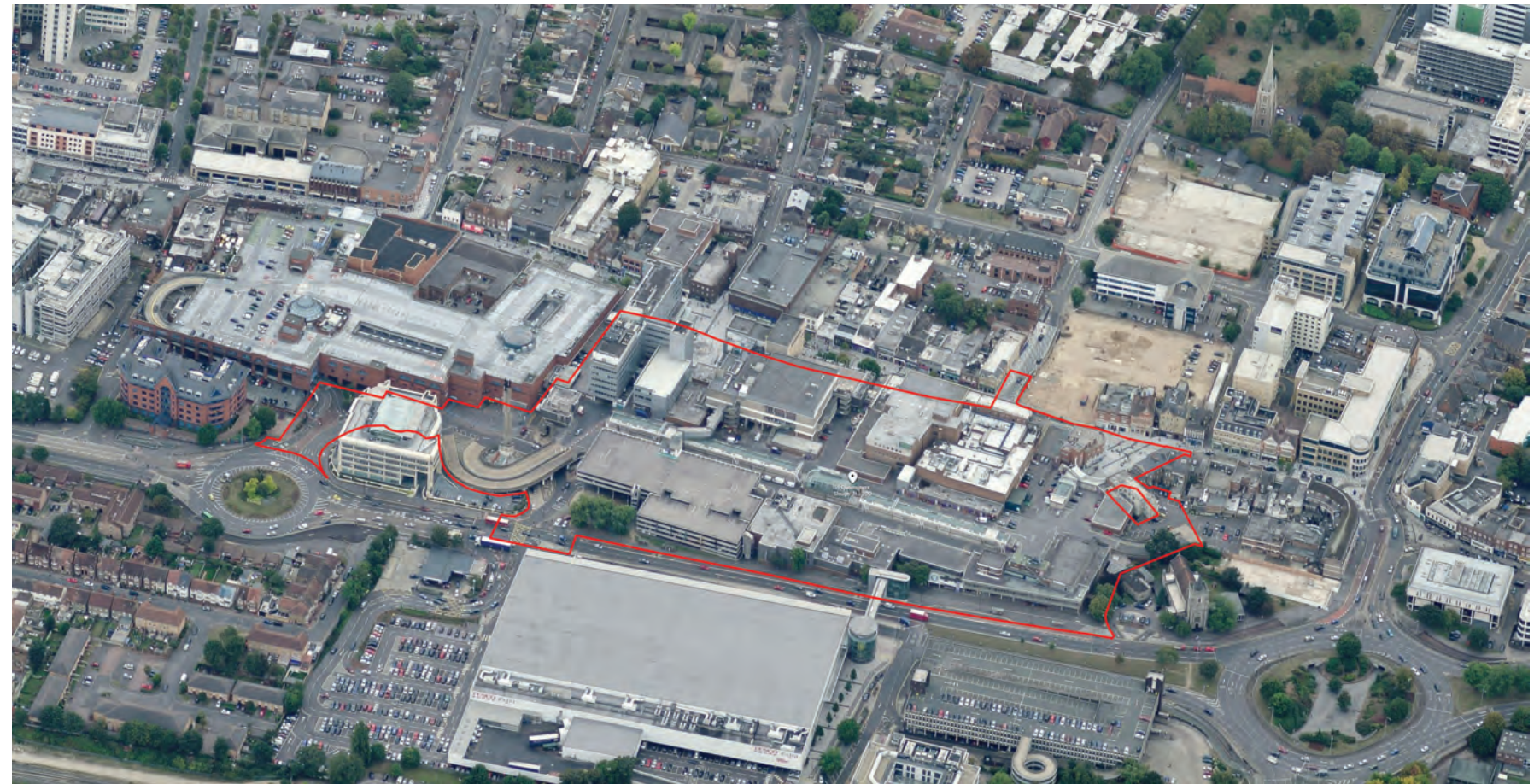
Fig. 5 - Existing aerial photograph of Queensmere & Observatory shopping centres
