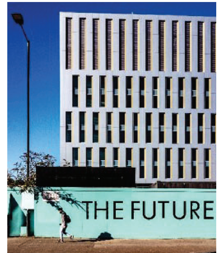
Fig. 35 - The Future Works, Slough - newly built office facilities
