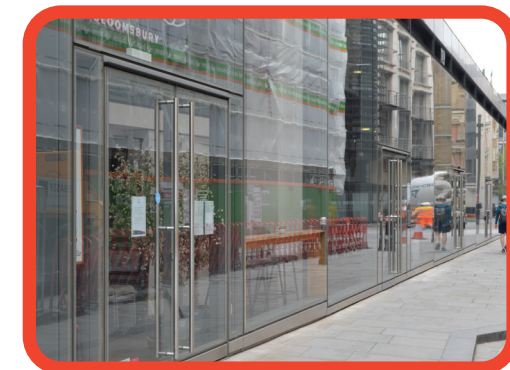
Lack of distinction and definition of retail units
