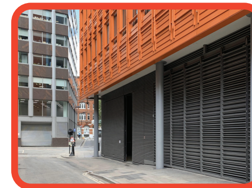
Prominent corner frontage occupied by plant room grilles
