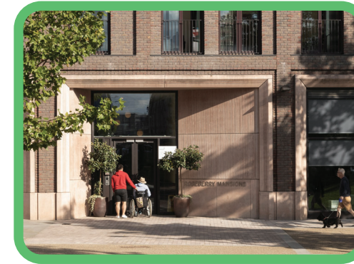
Level access and defined entrance doors
