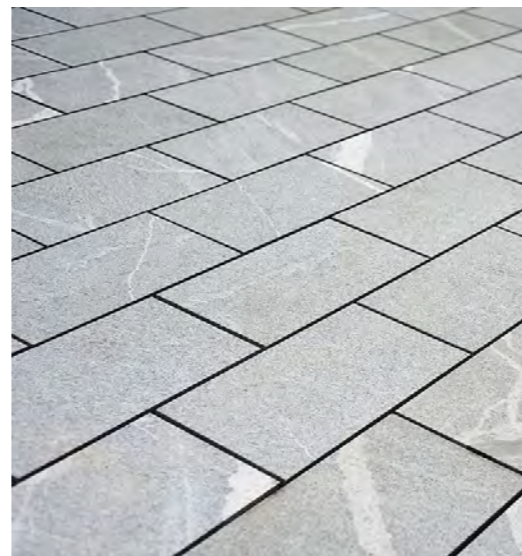
Material : Natural Stone paving Location: Town Square, lanes and streets Colour: mid/light grey
