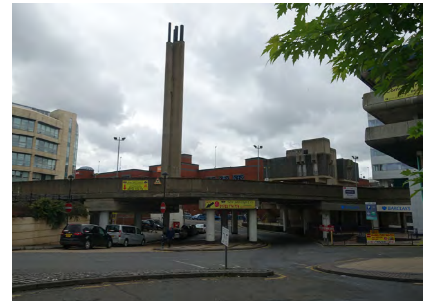
Fig. 20 - View of Queensmere Road site access & car park ramp
