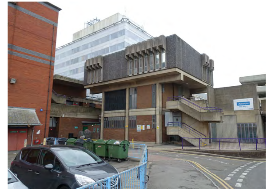
Fig. 25 - Vertical circulation to Queensmere car park
