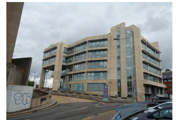
Fig. 53 - HTC office building
