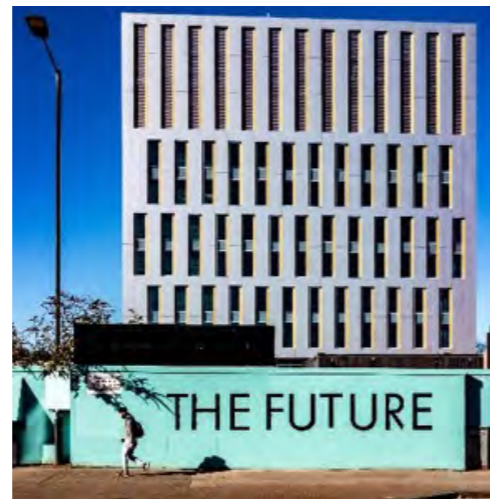
Fig. 88 The Future Works, Slough - office facilities
