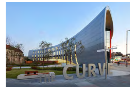
1. The Curve, Library and Cultural Centre.
