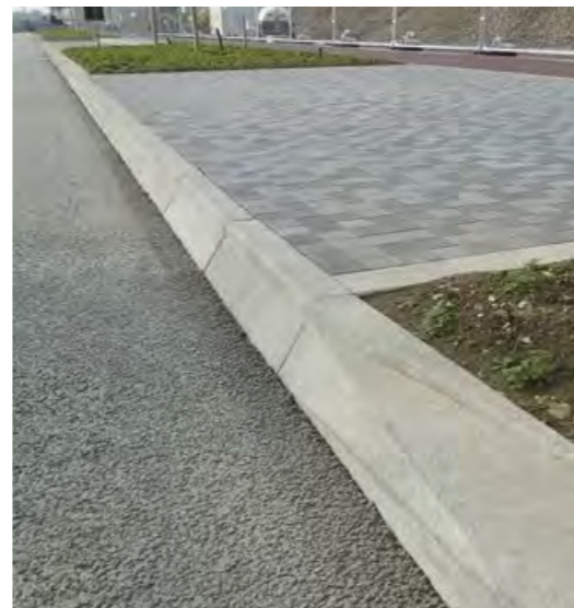
Material : Concrete Kerbs Location: Boulevard carriageway Colour: Mid grey
