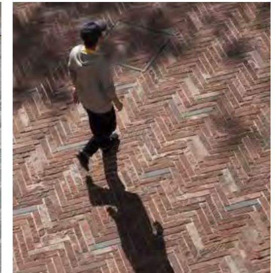
Material : Feature Dutch Clay Brick Pavers Location: Feature Seating Spaces Colour: Brown/Red
