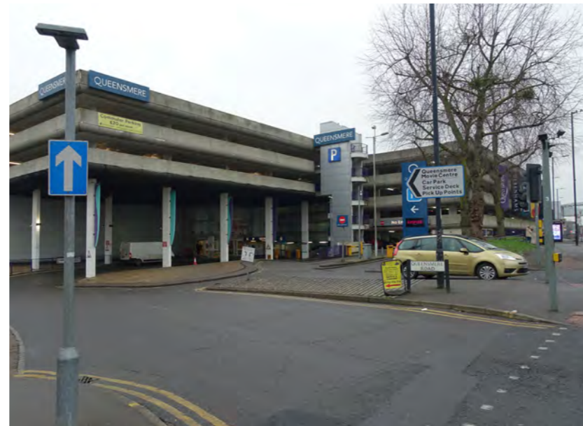
Fig. 24 - Queensmere multi storey car park on Wellington Street
