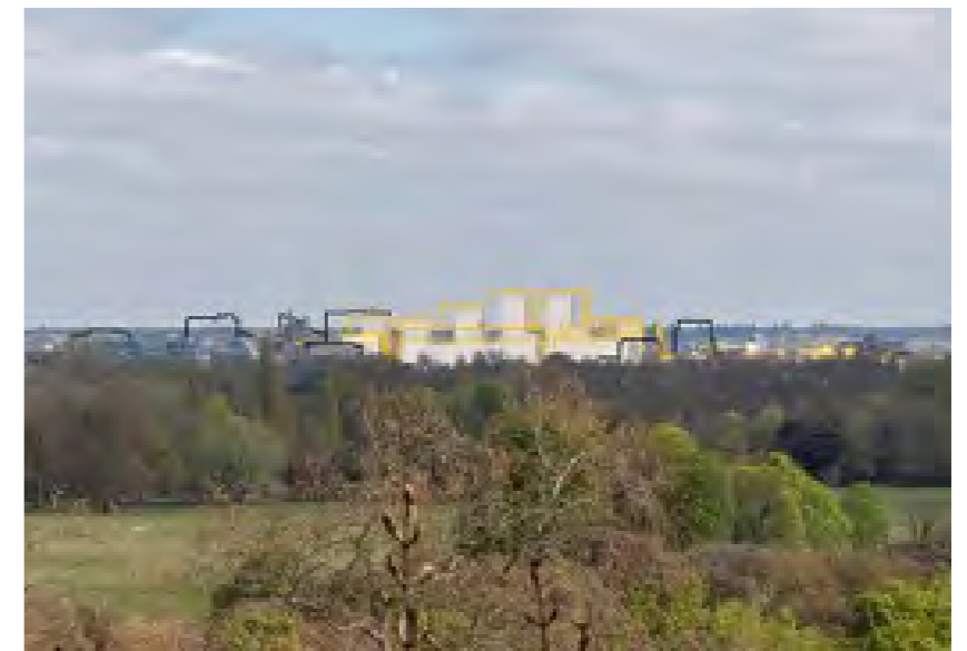
Fig. 134 - Testing of maximum parameters massing in long distance views (please refer to TVIA)
