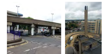
8 & 9. Carpark ramp/ Chimney
